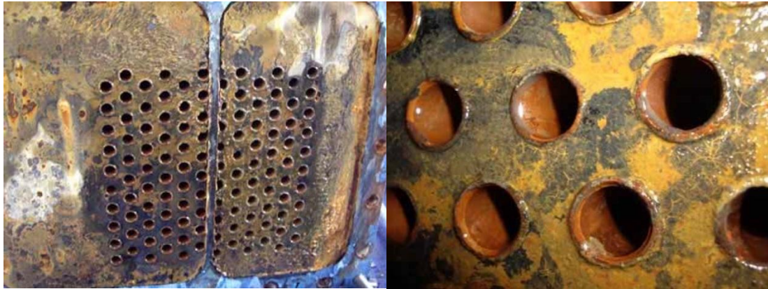
The inside of the heat exchanger (left) and a magnified view of the pipes (right).
