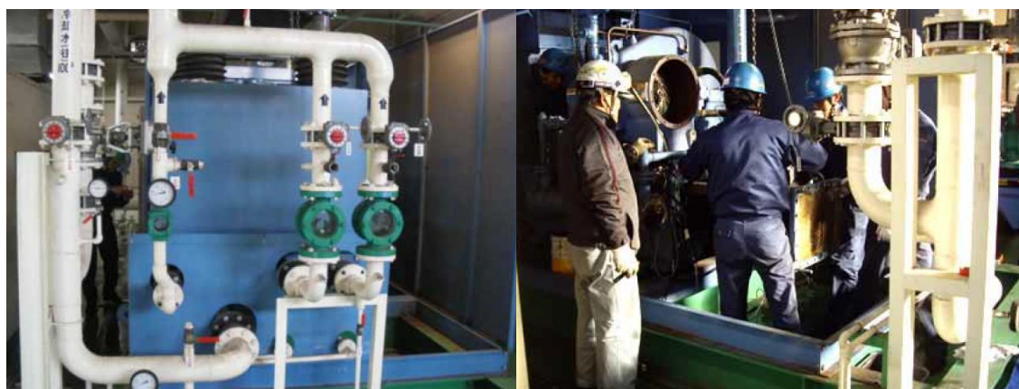
No. 3 Compressor front view (left) and engineers disassembling the compressor (right)
